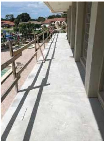
*Preparations are being made for the MBS Waterproof deck coating system on the balcony.*
