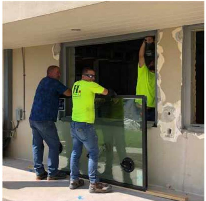
*The first of the new windows being installed in the renovation are going into the expanded Fitness Center.*
